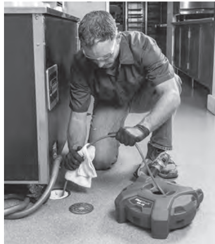
Figure 15 – Applying Lubricant to the Cable Sheath
